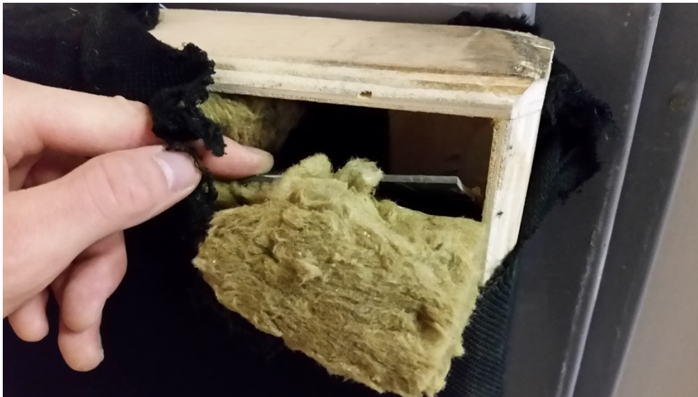
Figure 4 – Detail of the insulated core.
